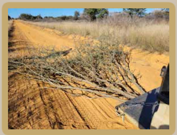
Truck used to drag the road.
